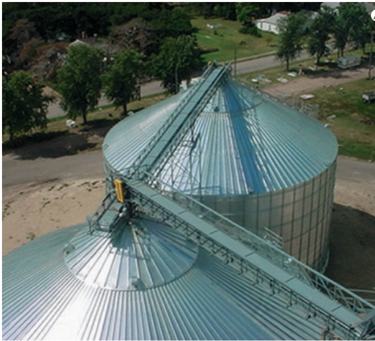
A Bin wall and roof are strong enough to carry required equipment and conveyor loads B Heavy-duty wall stiffeners provide extra strength C Anchor bolts at each stiffener secure the bin to the foundation D Variable Section Stiffeners (VSS) E Bolted connections and curved "Z" sections at roof transition provides tight, sealed connections F Curved tube supports and "Z" sections provide 100% contact and support to the roof panels with no gaps G The snug fitting inner and outer door combination provides a weather and grain seal
