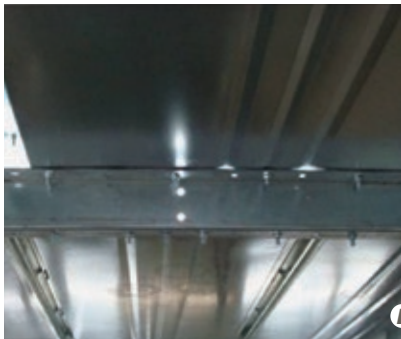
A Bin wall and roof are strong enough to carry required equipment and conveyor loads B Heavy-duty wall stiffeners provide extra strength C Anchor bolts at each stiffener secure the bin to the foundation D Variable Section Stiffeners (VSS) E Bolted connections and curved "Z" sections at roof transition provides tight, sealed connections F Curved tube supports and "Z" sections provide 100% contact and support to the roof panels with no gaps G The snug fitting inner and outer door combination provides a weather and grain seal
