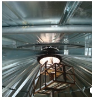
A Bin wall and roof are strong enough to carry required equipment and conveyor loads B Heavy-duty wall stiffeners provide extra strength C Anchor bolts at each stiffener secure the bin to the foundation D Variable Section Stiffeners (VSS) E Bolted connections and curved "Z" sections at roof transition provides tight, sealed connections F Curved tube supports and "Z" sections provide 100% contact and support to the roof panels with no gaps G The snug fitting inner and outer door combination provides a weather and grain seal
