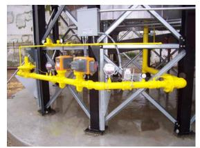
Commercial block and bleed gas train is standard with high & low gas safety pressure switches.
