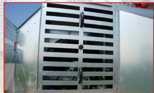
Lower Service Access Area
